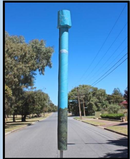
An example of how the tower could be shrouded and camouflaged
