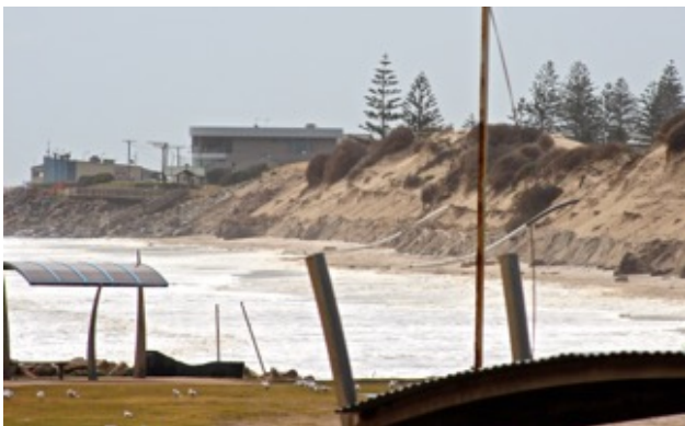
Coastal erosion with the West Beach SLSC under threat
