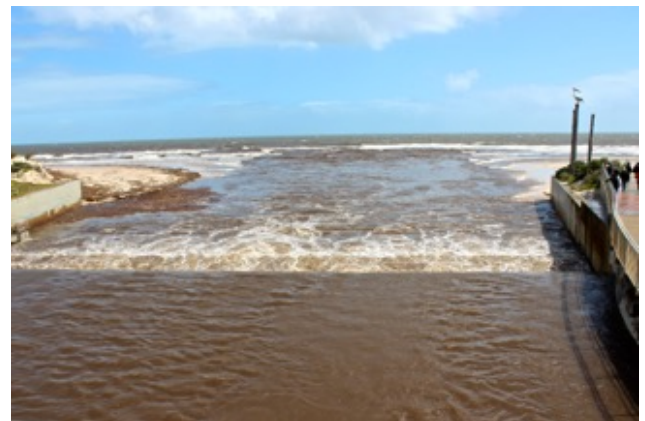
Polluted Storm water - Torrens River, Breakout Creek
